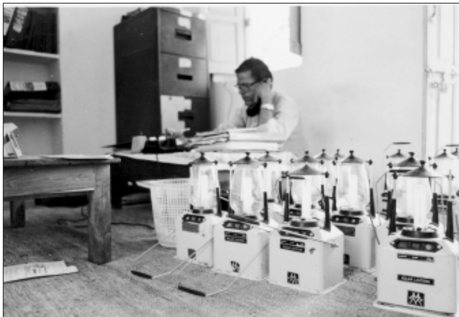
Photo 6. Barefoot solar engineer on solar-powered telephone exchange with 200 lines. Next to him are fabricated solar lanterns.
